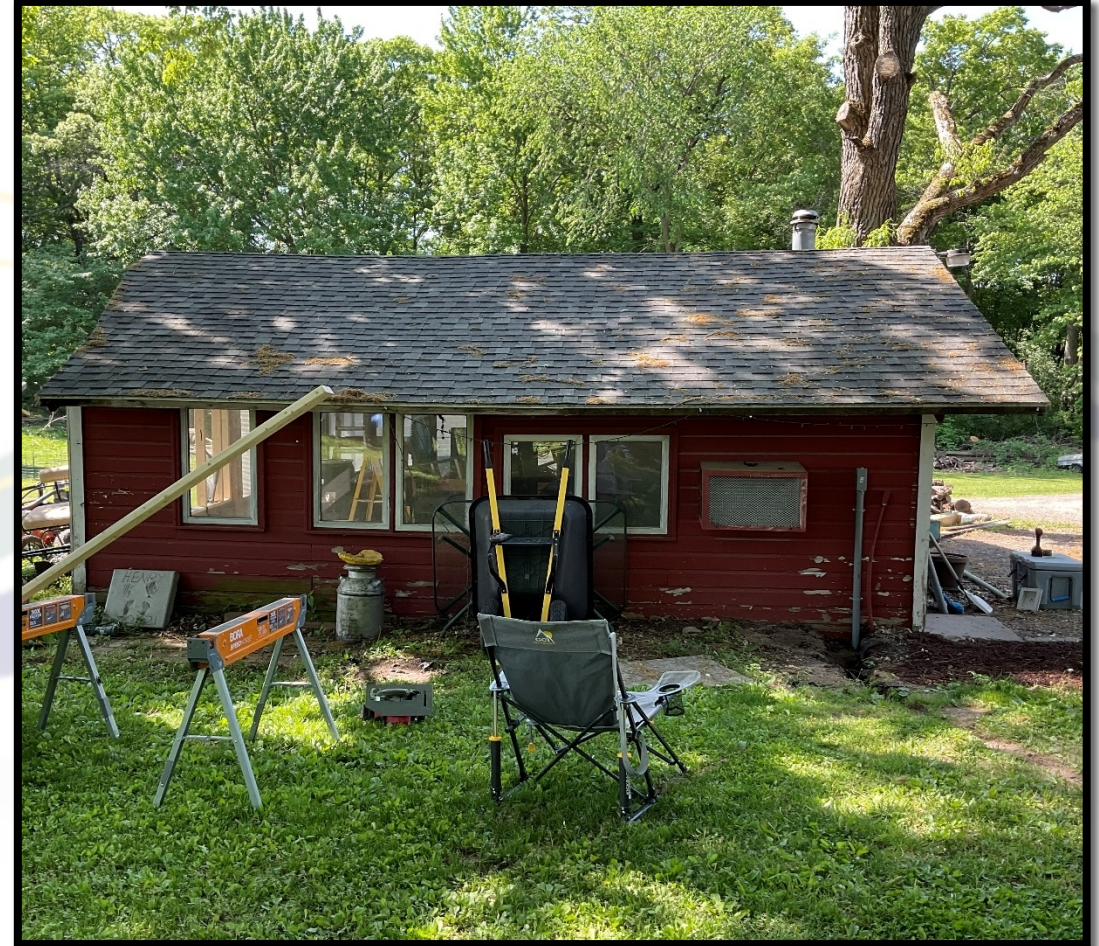
Accessory structure, looking south.
